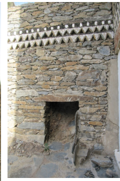
Figure 15. The entrances are at the same plane with the wall and decorated with marw stone
