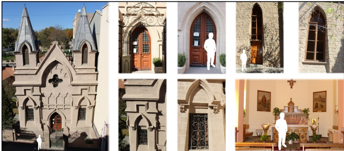
Figure 5: Photographs of the St. Paul Catholic Church
