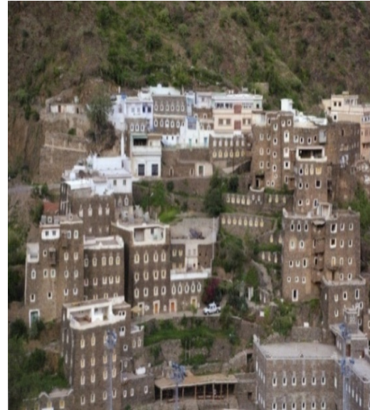
Figure 8. The urban fabric within the village of Rijal Al-Maa' is famous for its cohesive style of buildings
