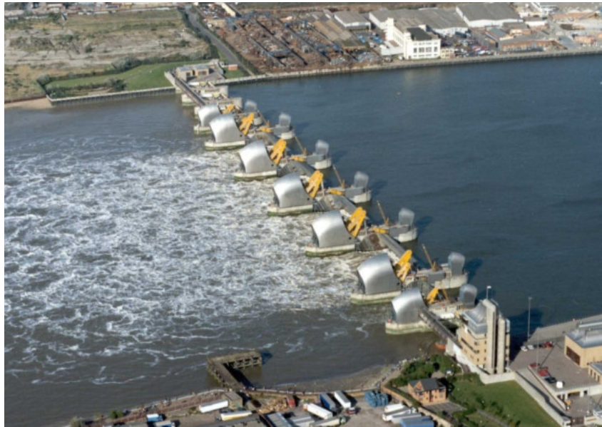
Figure 6. Thames Flood Barrier- London (Brooke, 2015).
