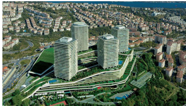
Figure 4: VRS implemented on podium level - Zorlu Center – Zincirlikuyu- Beşiktaş https://tr.onduline.com/tr/homeowner/kesfet/galeri/ondugreen (retrieved: 10.12.2019)
