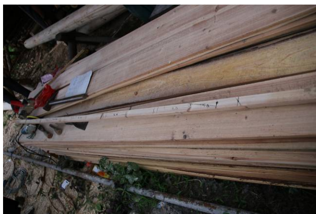
Figure 4. Dimension pole, photo taken from a construction site, Tongdao County, 12/08/2016 (木制杖杆, 拍摄于湖南通道某建筑工地)
