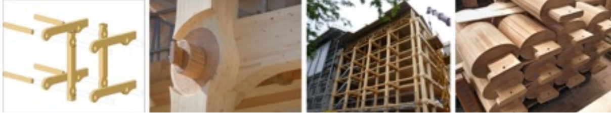
Figure 3:(a) Assembling Detail (b)Joinery Detail and (c)Tamedia office Building Wood Frame Structure (Shigeru Ban Architects 2013) (4) Wood joinery detail (Blumer-Lehmann AG 2014)
