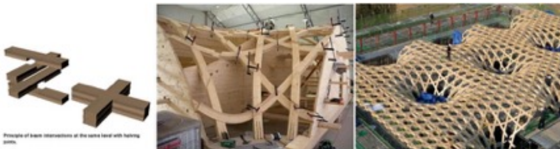
Figure 2: Scarf and halving joints for the Clubhouse's wood lattice structure, (Jeska et al. 2014, pp. 113,115,116)
