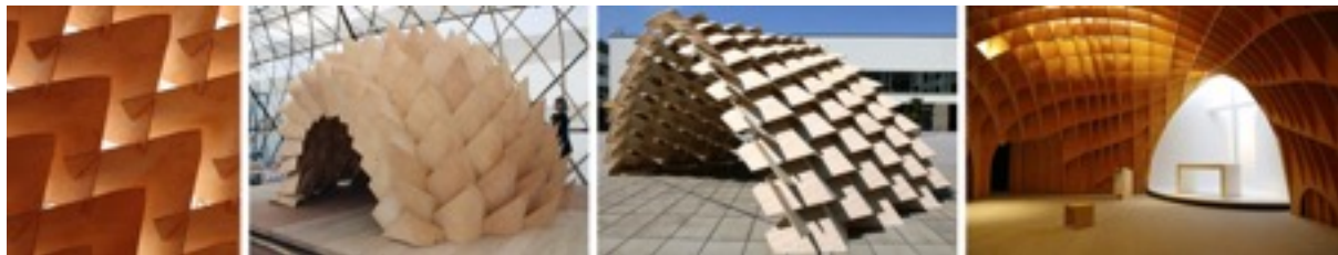
Figure 7: (a) Sliding slot joints-Dragon Skin Pavilion (b) dragon Skin Pavilion (Tynkkynen 2012) (c) IBOIS Prototype (Laboratory for Timber Construction IBOIS 2012) (d) and Autobahn Church (Schiffer 2013)
