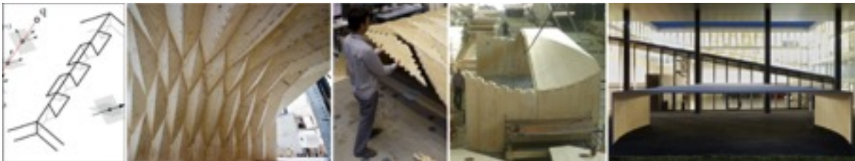
Figure 5: from left to right, (a) Interlocking Dovetail Joint illustration (b) Prototype 1 Folded plate shell (c) Prototype 1 during assembly (d) Prototype 2 during assembly (e) Prototype 2, spanning 13.5m (Robeller and Weinand 2015)
