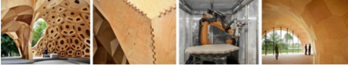
Figure 4: (a) ICD/ITKE 2011 Research Pavilion (b) Finger Joint Detail and (c) Robotic Fabrication of Plates (Institute for Computational Design 2011) (d) Landesgartenschau Exhibition Hall (Menges 2014)
